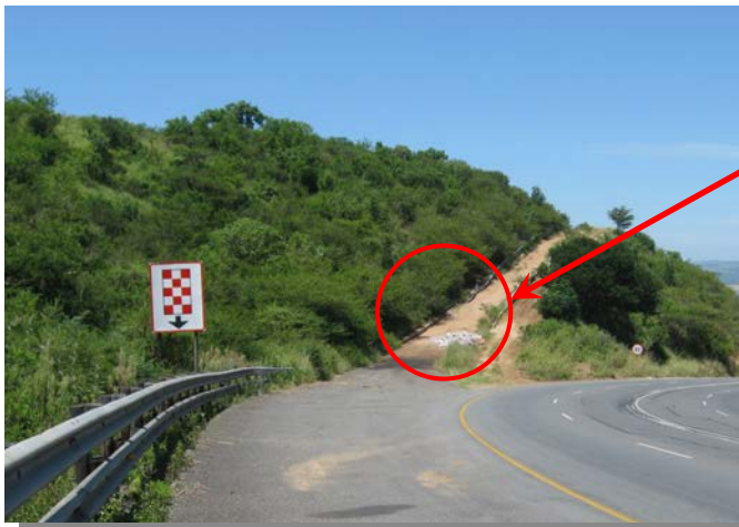
Truck arrestor beds need to be marked in a standardized way and should be kept clear of refuse and properly maintained to offer best functionality.
