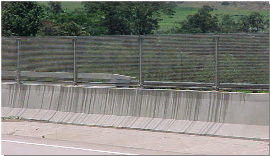
Glare screens erected on concrete barriers to reduce possible headlight glare.
