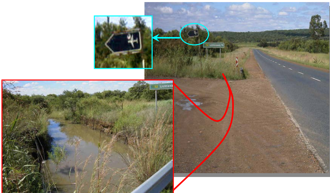
Although a short section of guard rail has been installed adjacent to the road, no protection is given for an errant vehicle using the gravel intersection on the left
