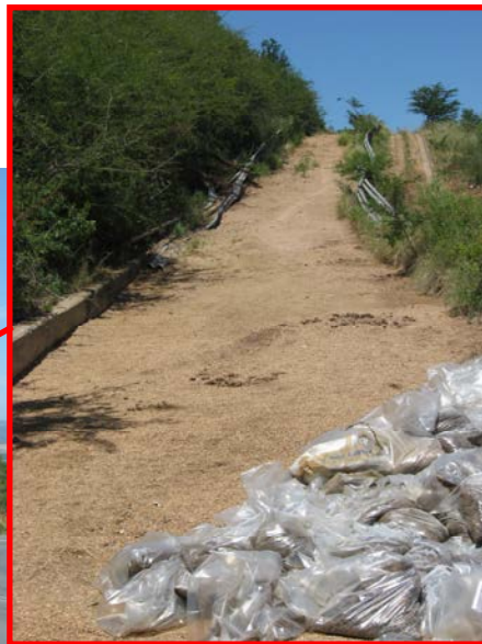
Truck arrestor beds need to be marked in a standardized way and should be kept clear of refuse and properly maintained to offer best functionality.
