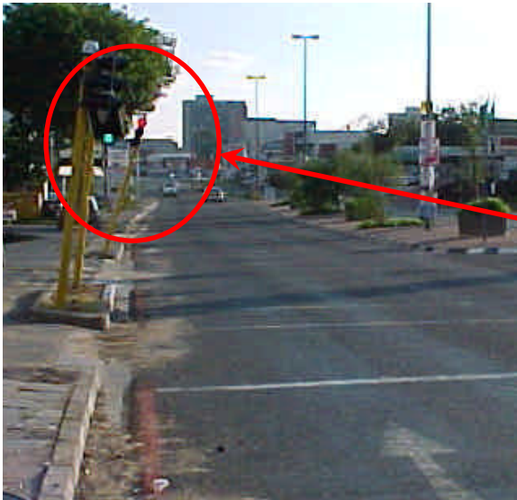
These signals had been damaged during a crash. Approaching motorists now simultaneously face RED and GREEN signals.
