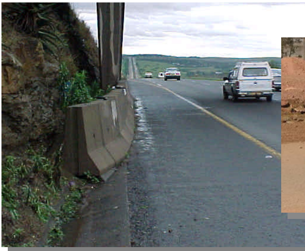
Traffic Barriers with no or inappropriate end treatment; The end-treatment is supposed to provide gradual energy dissipation in case of a crash.
