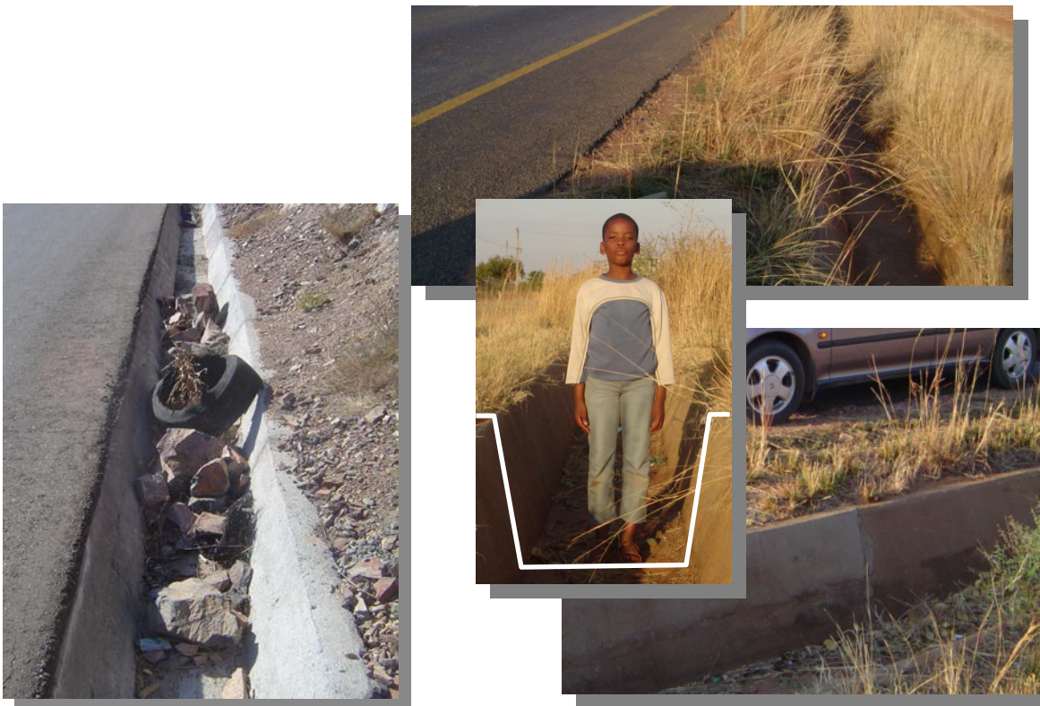
Non-recoverable drainage ditches
