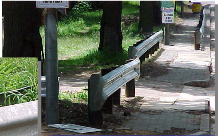
Short lengths of guardrail are hazardous because there is insufficient length to develop tension to counter the forces of a crash
