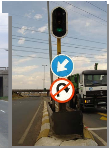
The efficient use of backboards to ensure contrast against a variable background
