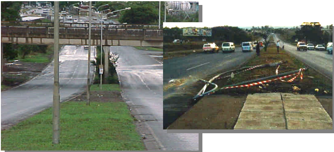
Unprotected lighting poles can pose a serious hazard to road users – as shown above.
