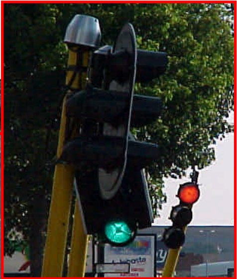
These signals had been damaged during a crash. Approaching motorists now simultaneously face RED and GREEN signals.
