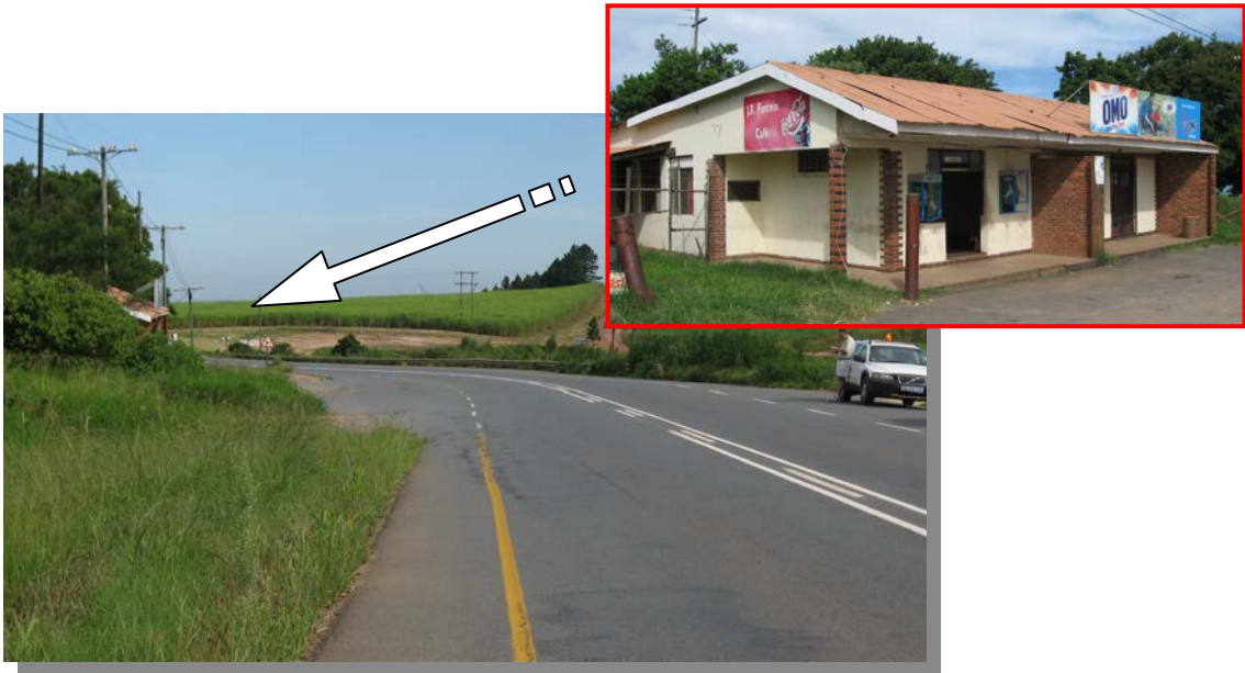
Hidden entrance to roadside store, located on a curve with restricted sight distance from both directions
