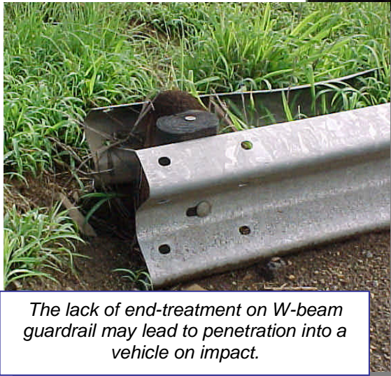
Short lengths of guardrail are hazardous because there is insufficient length to develop tension to counter the forces of a crash
