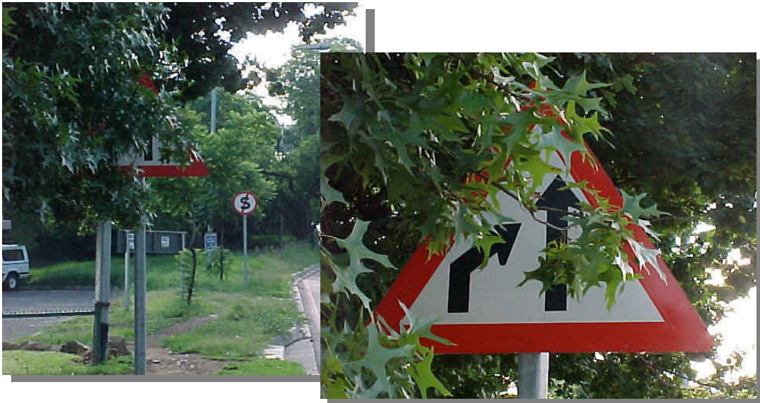
A Warning sign obscured by overgrown vegetation
